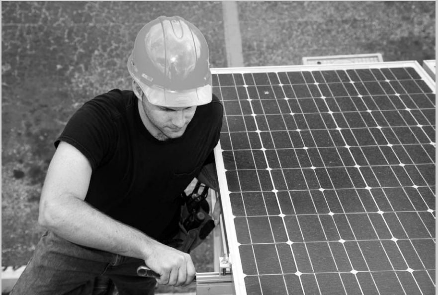
An electrician installs solar panels on the side of a building.
