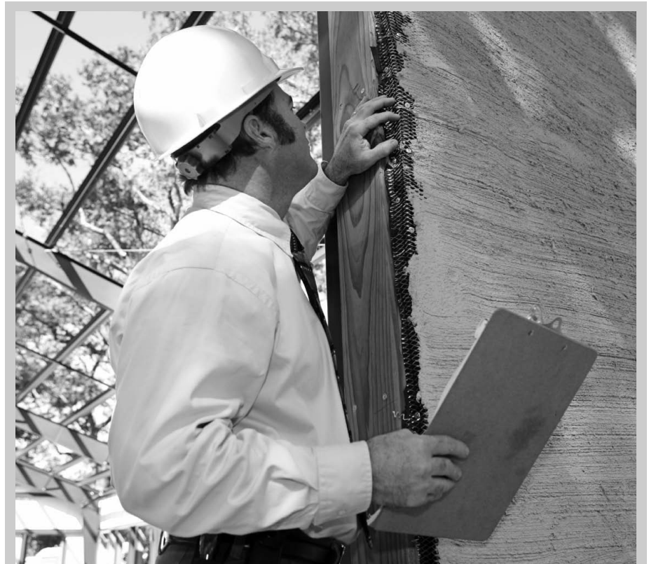
A building inspector checks over incomplete stucco work on new construction.
